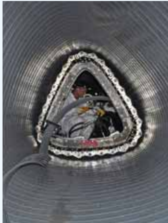
sewer and formed into a watertight pipe inside the old pipe.
